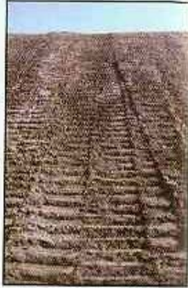
Rough graded or terraced slopes help keep soil in place.
